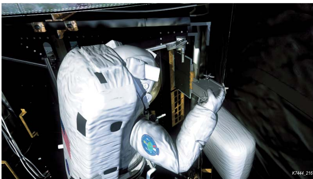
Fig. 2-15 John Grunsfeld carefully removes the first of two failed circuit cards from the Advanced Camera for Surveys. New cards will be installed and a power supply module attached to return the instrument to operation.
